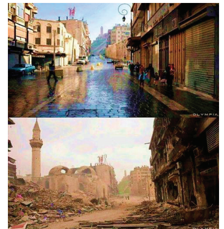
Figure 102: one of the main road to the citadel.
