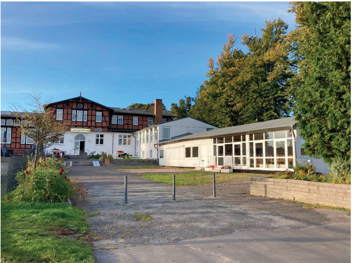
Figure 16: Access to the ferry house
