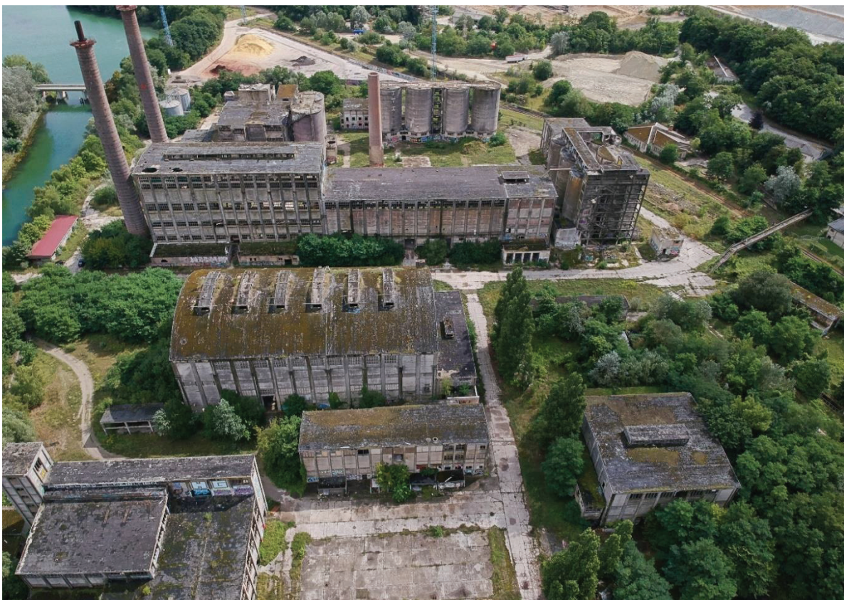
Pic 13 Buildings in the design area from bird eye view( AIV-Berlin-Brandenburg, 2021, no page)
