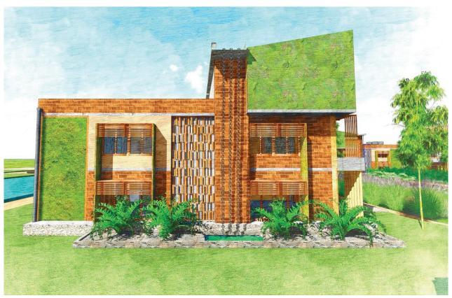
Side elevation of the house comprises of various elements to keep the house well ventilated and cool. Trellis on the southern side, rain chains leading the water to the sump, Clay jaali along the internal courtyard and wall creepers for insulation.
