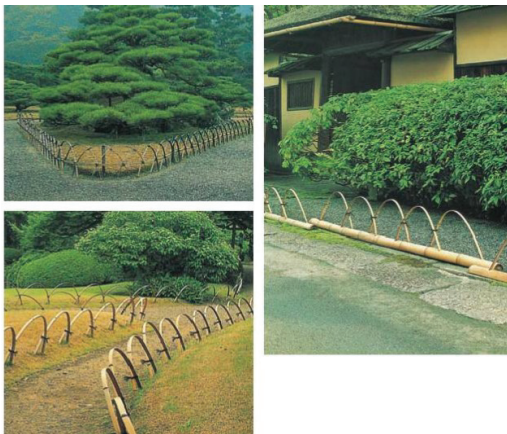
Figure 2.31: Type of bamboo fence –Nanako (Source: Yoshikawa Isao. Suzuki Osamu.2009. Bamboo fences.Princeton Architectural Press. Pp106-7)
