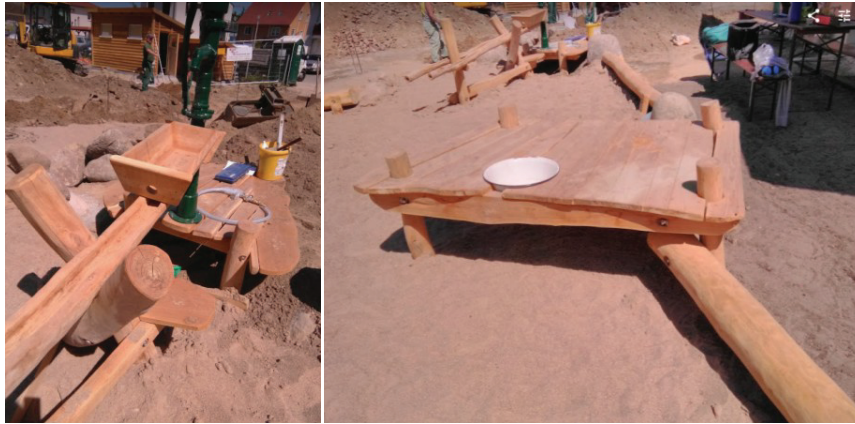
Figure 3.5: Playing pump for water play construction (Source: Personal archive)
