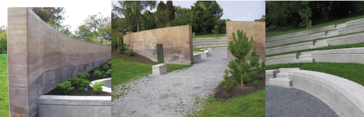
Figure 2.21: Rammed earth Amphitheatre at the UBC Botanical Garden-Vancouver Canada, Project 2010 by Forma Design (Source: http://rammedearth.blogspot.com/2010_09_01_archive.html )
