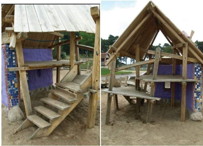
Figure L: Details of play equipment made of wood, tiles, and concrete. (Source: personal archive of Fiedler Sabine)
