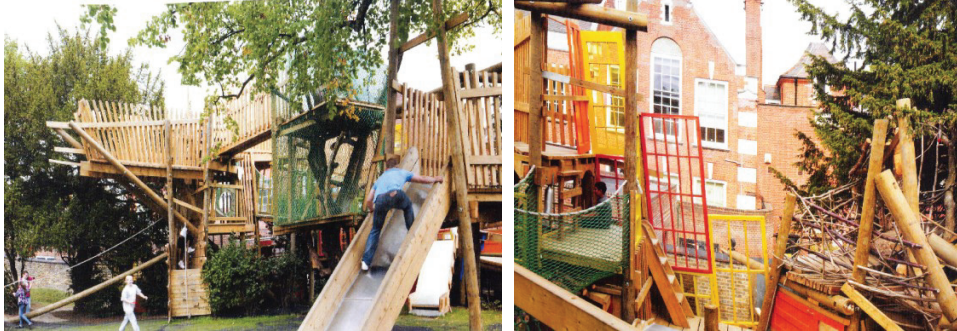
Figure 3.22: Kilburn Grange Park Play Center and Park, London by Erect Architecture Company Zurich (Source: Galindo.2012.p108.Playground Design.ISBN 978-3-03768-109-1.)
