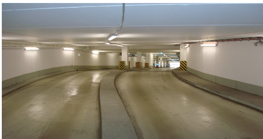
Figure 18 The Entrance of the underground parking
