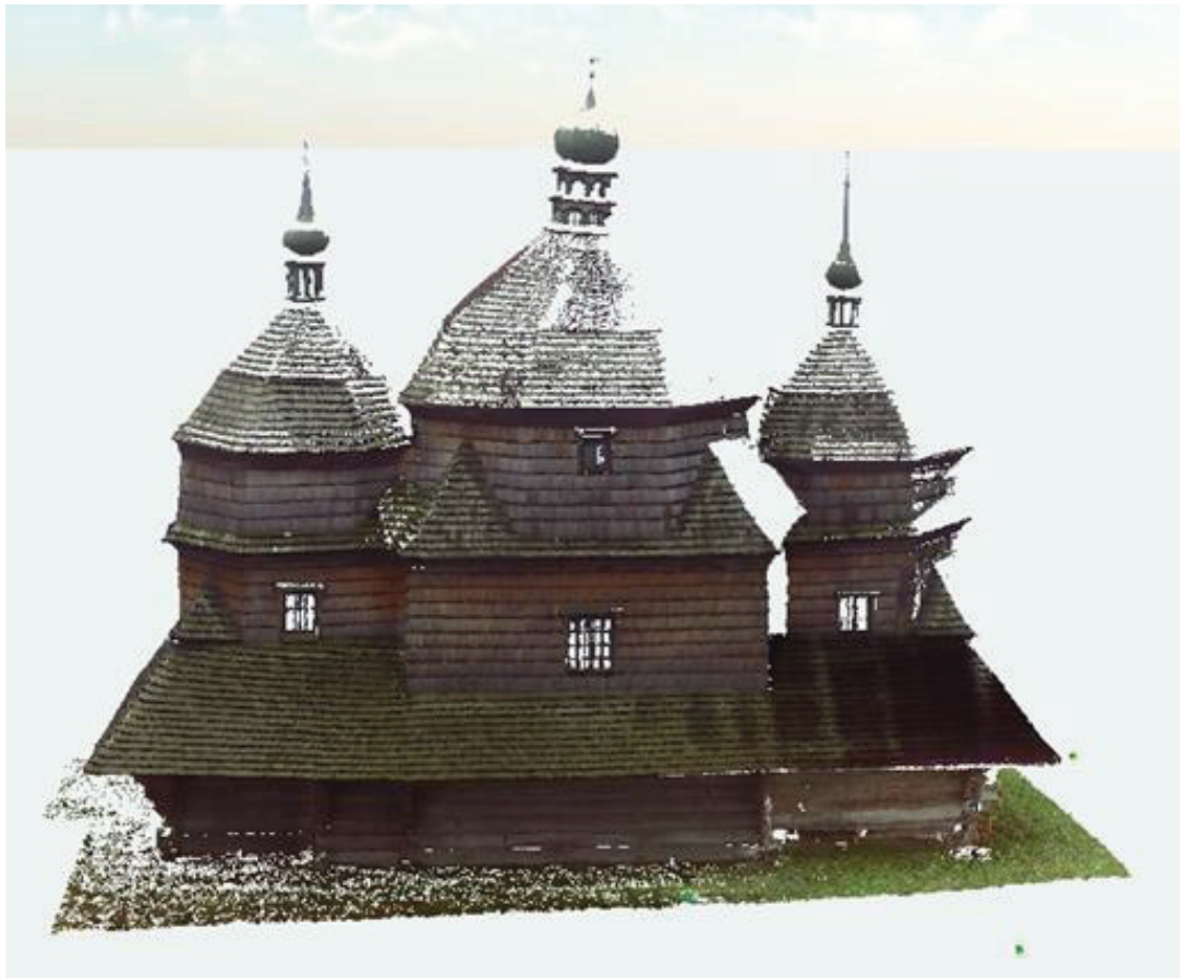
Figure 4.4: Point cloud of St. Archangel Michael church
