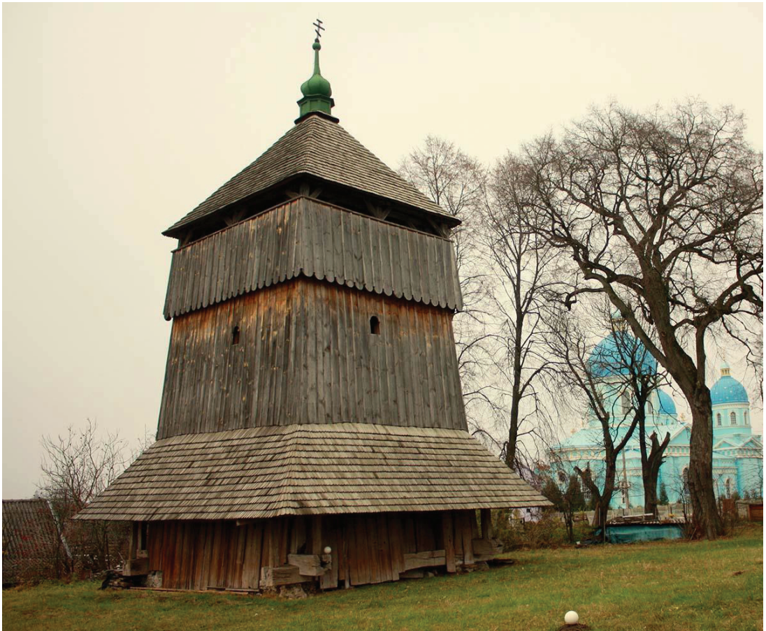
Figure 3.2: The Bell Tower
